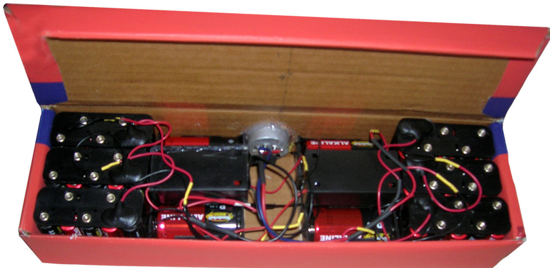
Photo 3b. Alternate battery layout using 60AA batteries in place of the ten 9 volt batteries. The dial light D cell is omitted due to space limitations, but you can purchase my Z-1 replica 1.5v cell to power the dial light circuit of 600 series or the filament string in the 8G005 series.
